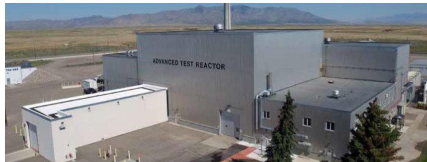
INL's Advanced Test Reactor (ATR)
